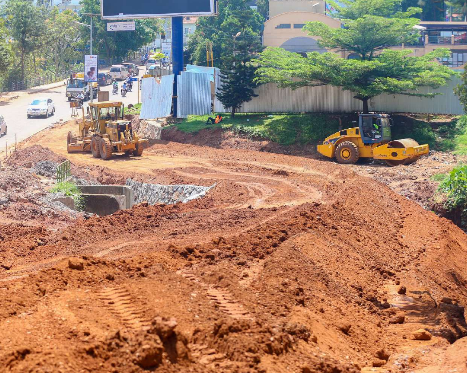
On going road works in Kampala
