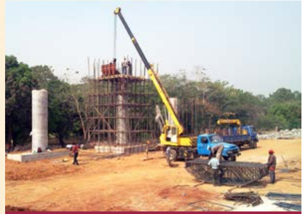
Construction in progress
