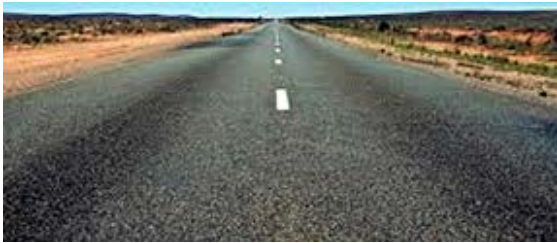
Fig. 2: First highway paved with recycled plastic in Mexico
