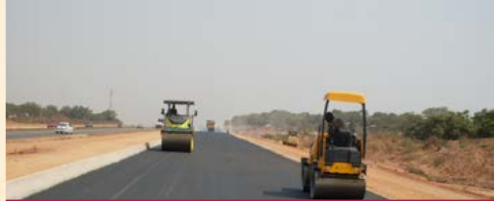
Outer Northern Express Abuja -laying and compaction of binder course
