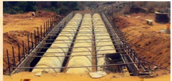
Construction in progress
