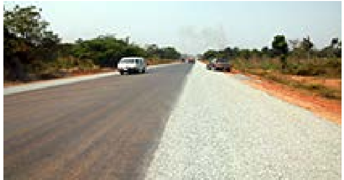
Fig. 4: A 2-lane single carriageway, a federal road continuity in rural areas
