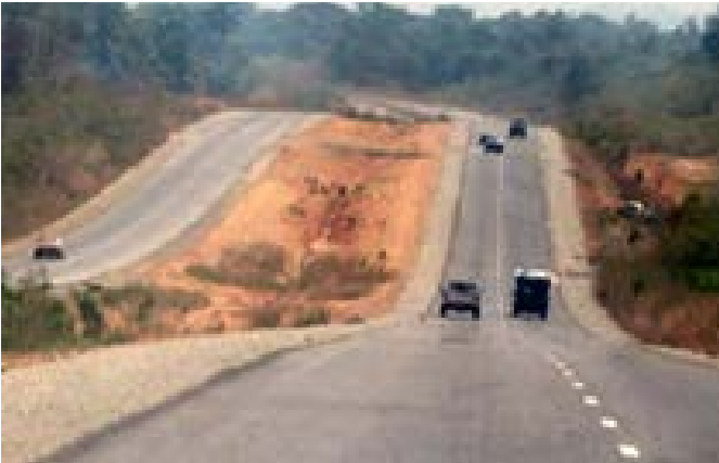
Fig. 3: A dual carriageway for a road network
