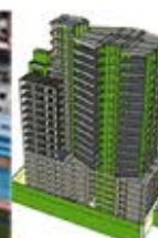
Ocean Heights (Twin tower) in Lagos.
