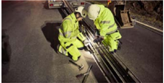
Fig. 6: A road-embedded power line being constructed
