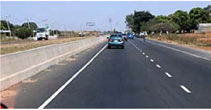
Fig. 1: A Dual carriageway with concrete crash
