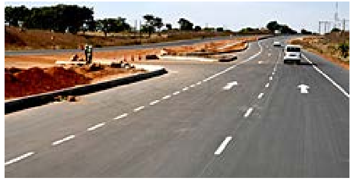
Fig. 2: A freeway with control of access and median
