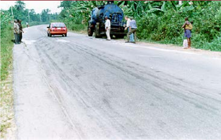
Port-Harcourt - Warri Road Rehabilitation
