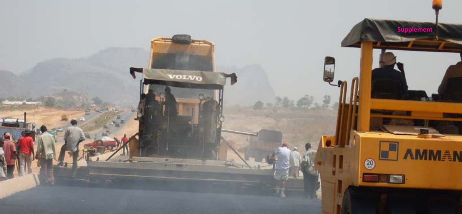
Outer Northern Express Abuja-Compacting binder course
