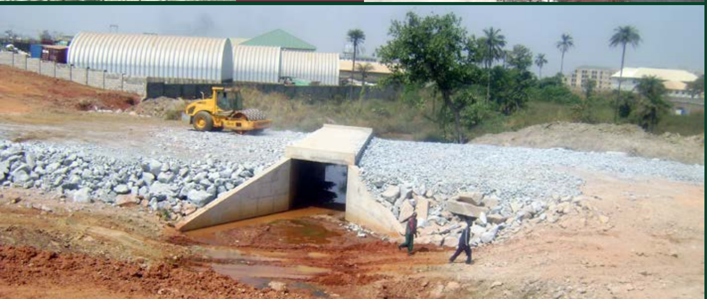
Construction in progress
