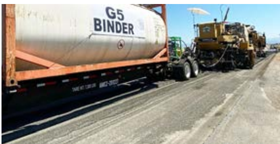
Fig. 3: California highway paved with plastic
