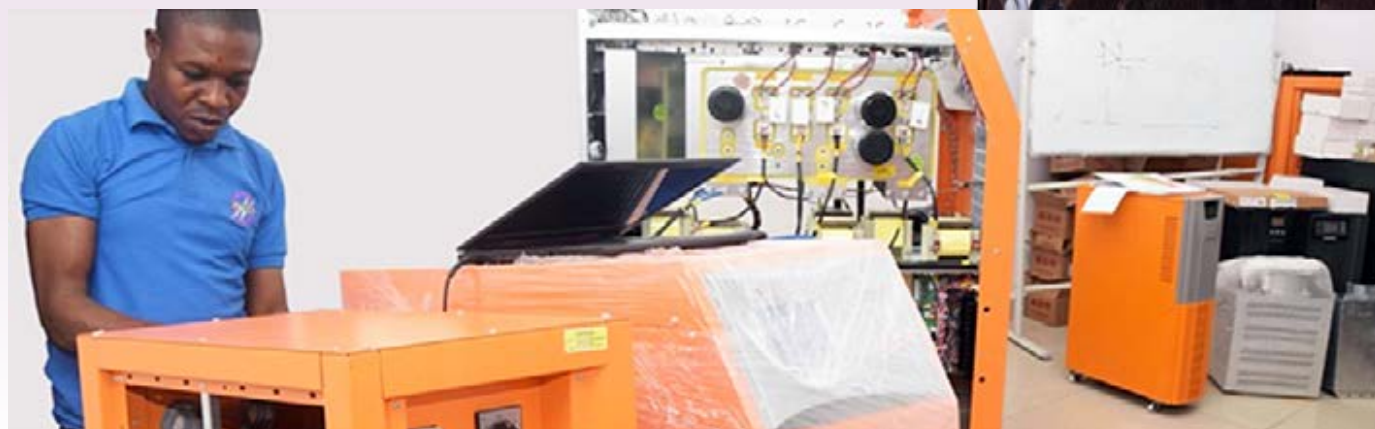
A staff working on an Uninterruptible Power Supply, UPS, system
