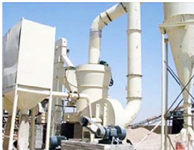
Fig. 3: Barites processing plant
