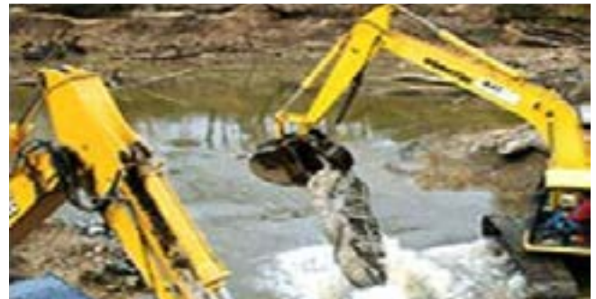
Fig. 2: Heavy dam construction equipment
