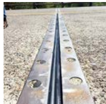
Fig. 13: A completed joint
