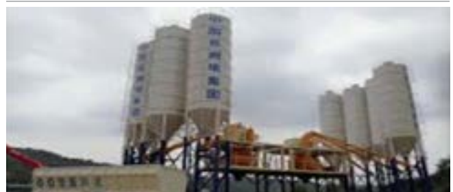
Fig. 3: Concrete batching plant
