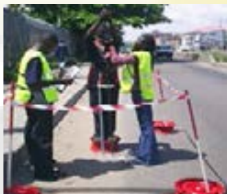
Pavement Evaluation in progress: Dynamic Cone Penetration
