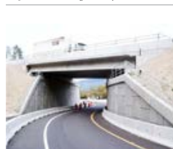
Fig. 14: Retaining walls (wing walls) in front of abutment supports
