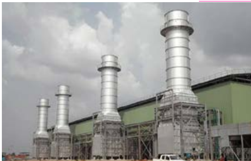
A thermal power plant in Southeast Nigeria
