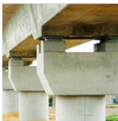
Fig. 7: A pot bearing
