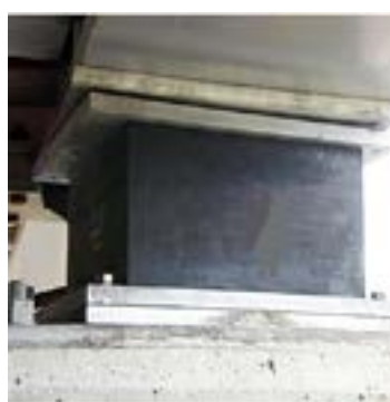
Fig. 9: A neoprene bearing
