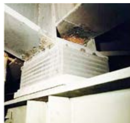
Fig. 8: An elastomeric bearing
