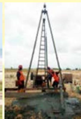
Percussion drilling in progress
