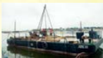
Off Shore drilling - Percussion Drilling from the top
