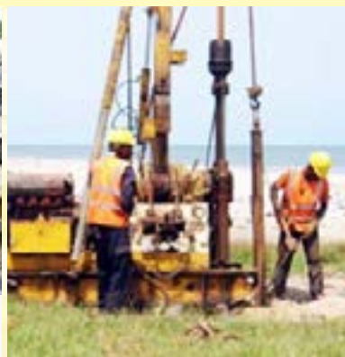
Crew at work using Rotary Drilling usually for rock
