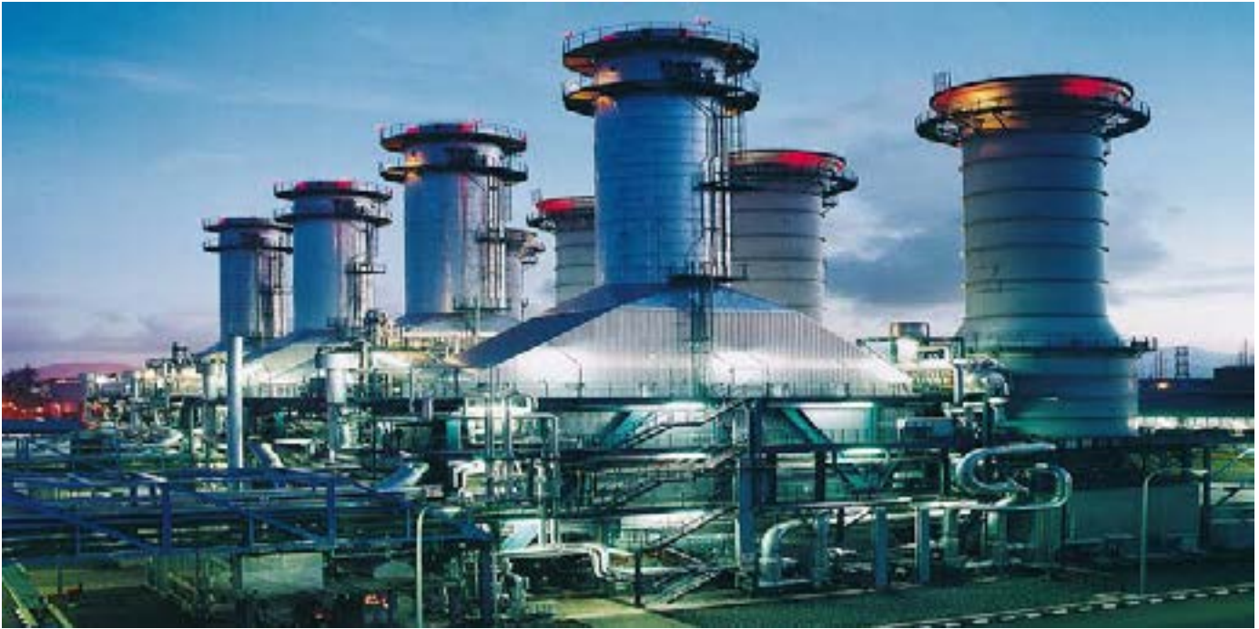
A thermal power generation plant in Nigeria
