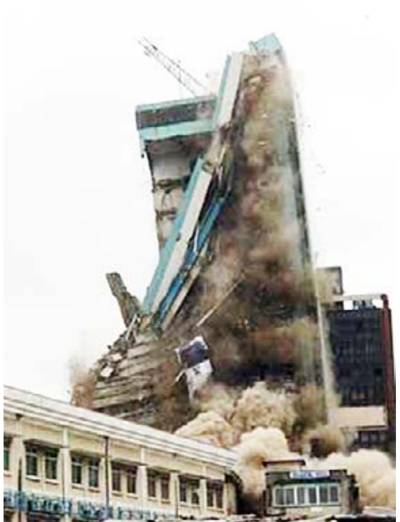
Fig. 2: The Bank of Industry building under demolition
