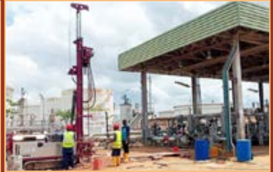
Geotechnical investigation at Kaduna Refinery
