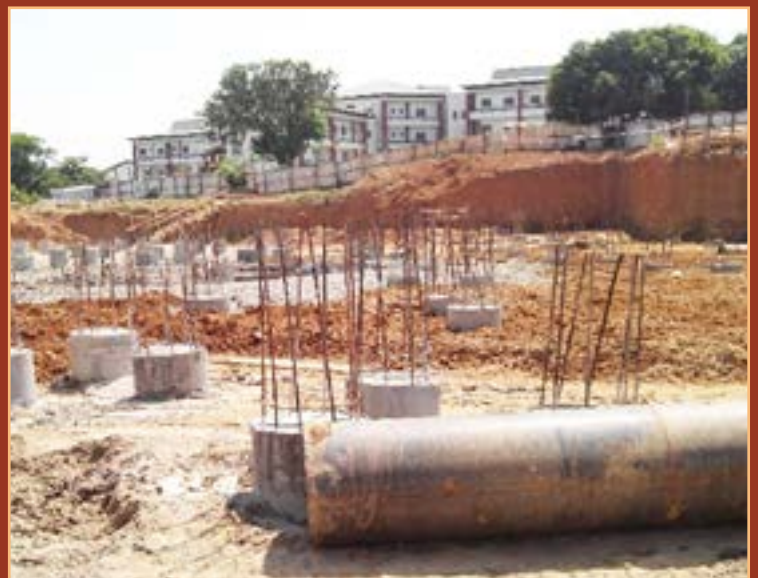
Pile works at National Hospital, Abuja
