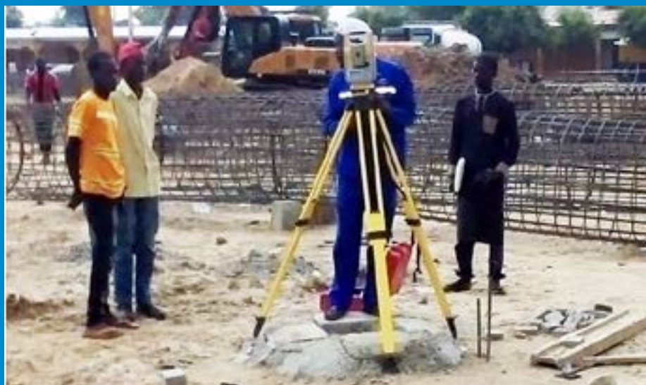
Surveying team at work
