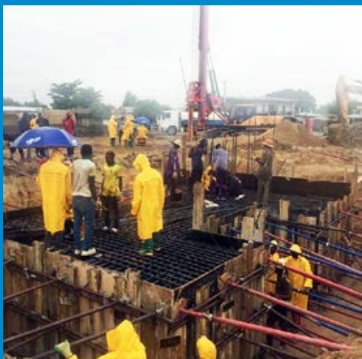
Ready to receive concrete
