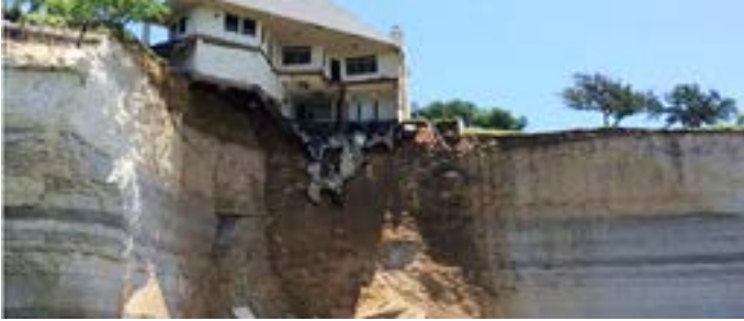
Fig. 4: A limestone bluff failure in Lake Whitney in Texas in 2014 (Source: https://www.capitalgeotechnical.com/geotechnical-failures.html )
