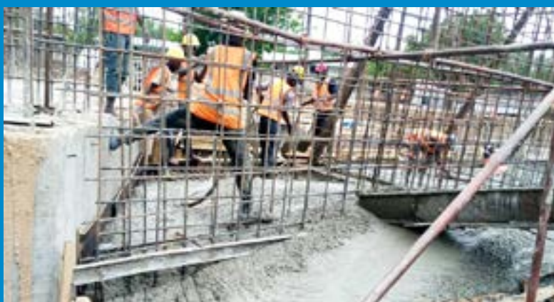
Casting of base for retaining wall
