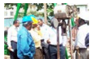
Figs. 6a and 6b: A typical set of drilling equipment for onshore geotechnical investigation
