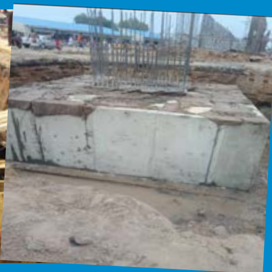
Cast r.c pile cap (5.5m x 8m x 2m)
