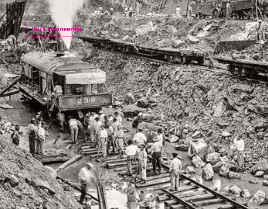
Fig. 1: Construction of Panama Canal. Picture (Source: Google image)
