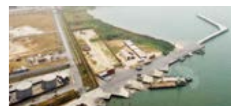
Fig. 2: Material Offloading Jetty 2
