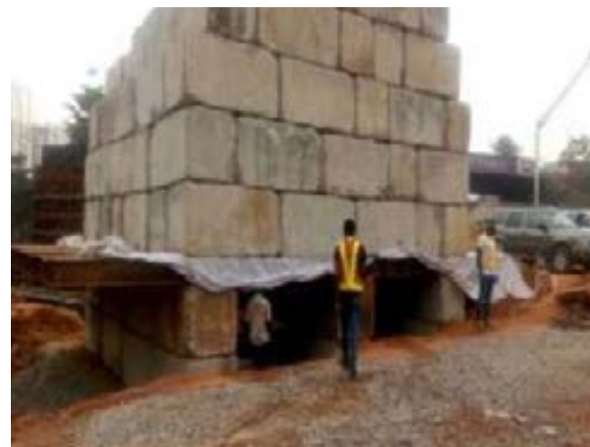
Fig. 7: A pile load testing for QAQC monitoring, Kentledge Method
