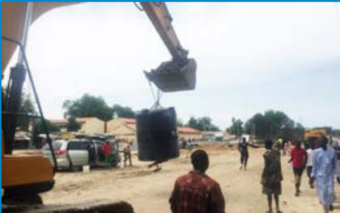
Preparation for pile load test
