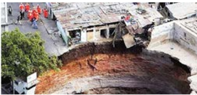
Fig. 5: A massive sinkhole in Guatemala in 2007 (Source: Ibid)
