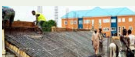
Construction of Indoor Sports Hall
