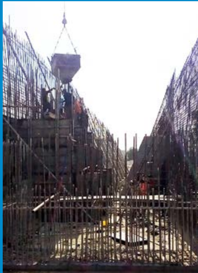
Casting of counterfort wall
