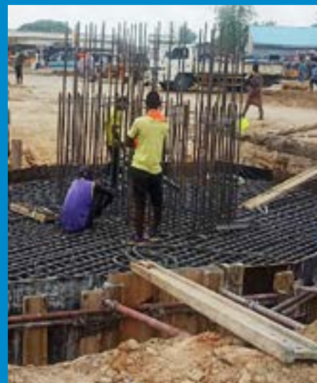
Pile cap ready for concreting
