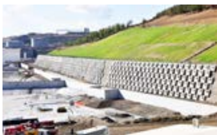
Fig. 5: A ground anchor installation site
