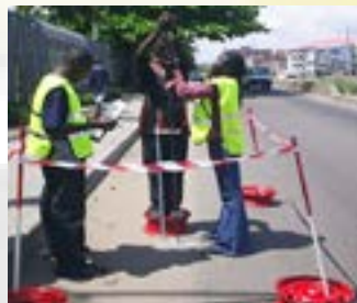
Pavement Evaluation in progress: Dynamic Cone Penetration
