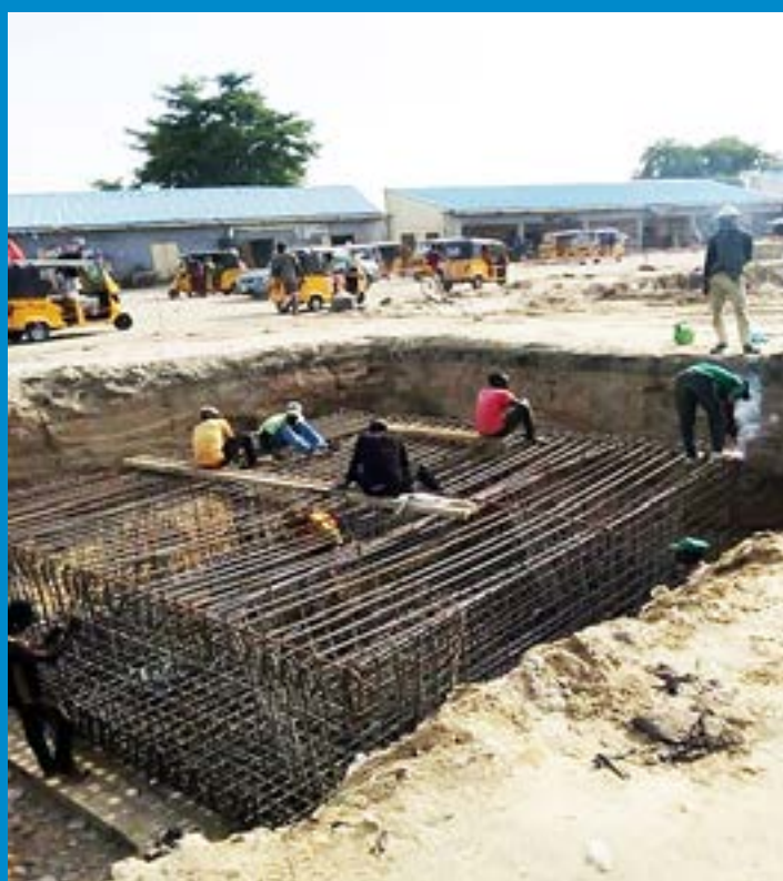
Re-bar arrangement for pile cap
