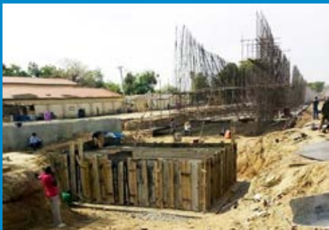
Formwork for Pile Cap
