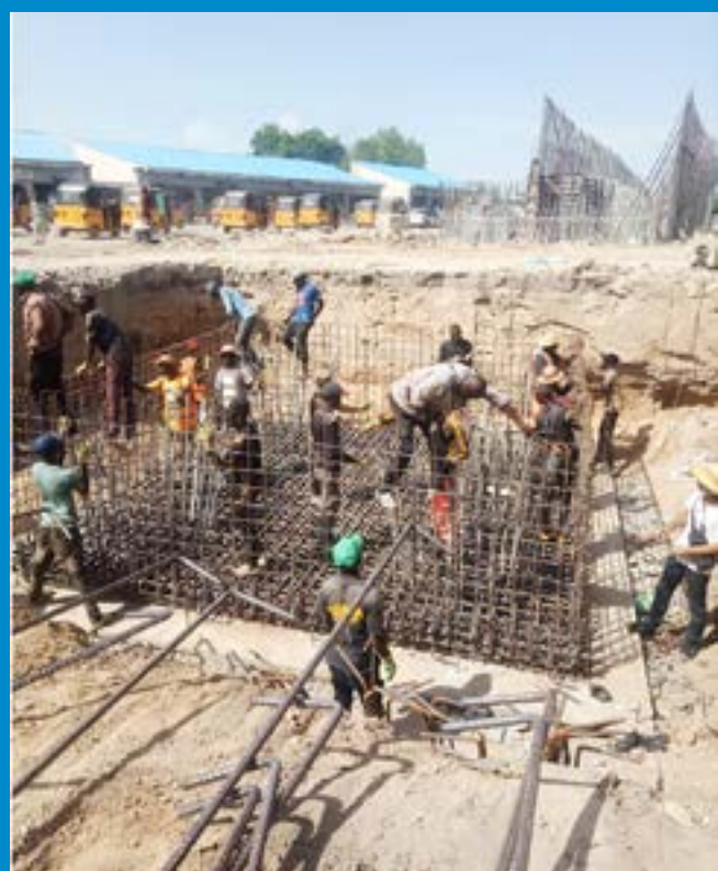
Re-bar arrangement for pile cap
