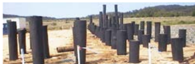
Fig. 8: A pile foundation construction in progress
