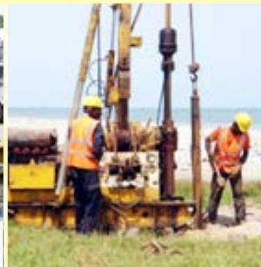
Crew at work using Rotary Drilling usually for rock
