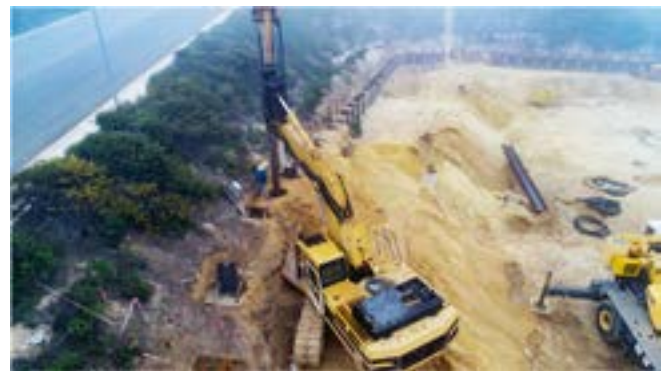
Fig. 7: Soldier piles installation site
