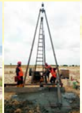
Percussion drilling in progress
