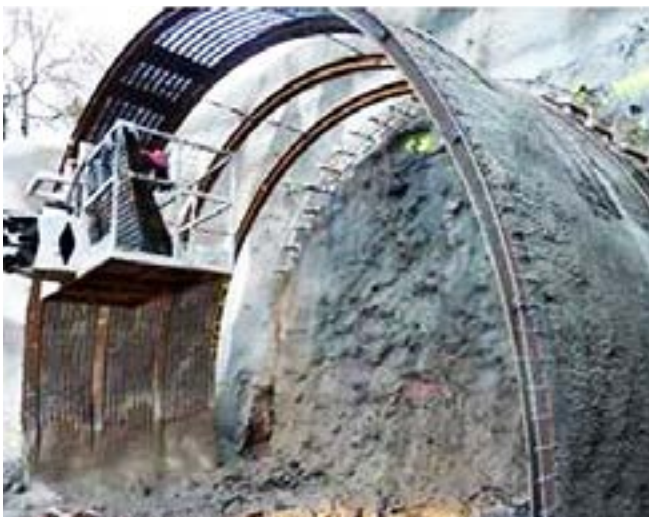
Fig. 3: A rock reinforcement and support (Source: Google Image)
