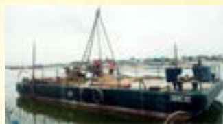
Off Shore drilling - Percussion Drilling from the top
