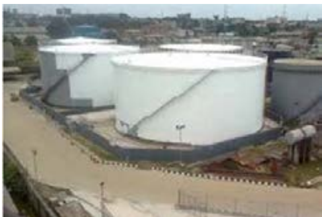
Fig. 6: An oil tank farm for downstream operations (Source: cakasang.com)
