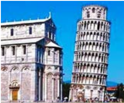
Fig. 4: The Leaning Tower of Pisa, Italy (Before restoration) – caused by unidentified weak soil layer at initial construction phase
