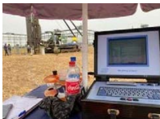
Fig. 8: A digital pile load testing (using a Load Analyzer)
