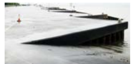
Fig. 1: An existing quay deck
