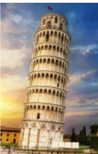
Fig. 6: The Leaning Tower of Pisa
