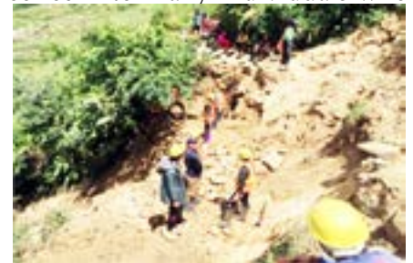
Fig. 3: Engineers on a landslide site
