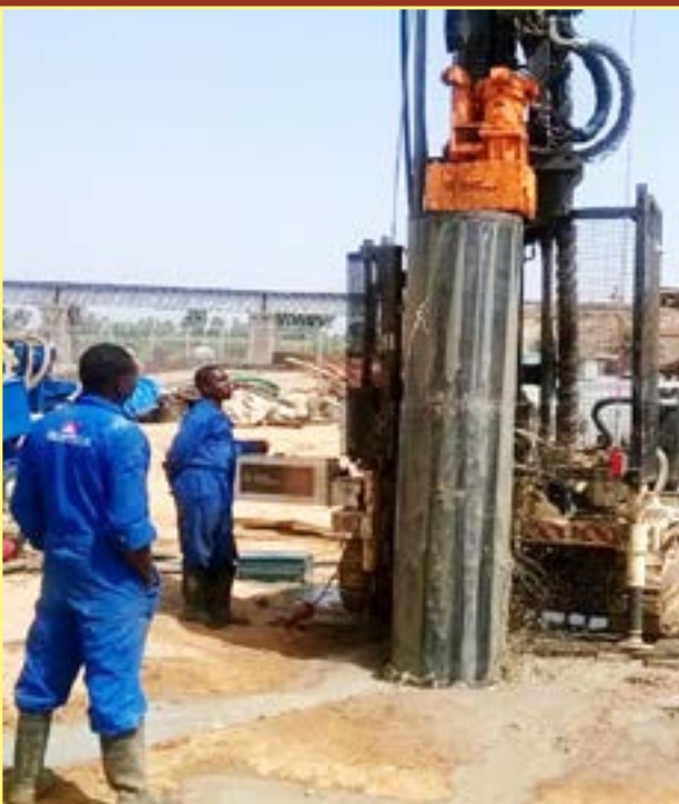
Pile construction at a project site
