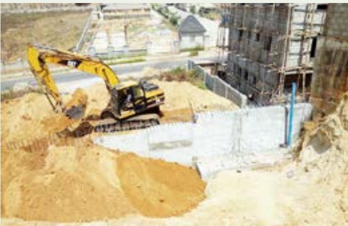
Construction 6M High Retaining Wall at Guzape District, Abuja
