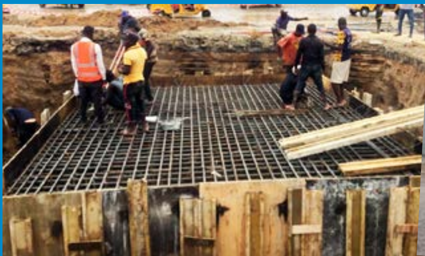
Formwork/re-bar arrangement
