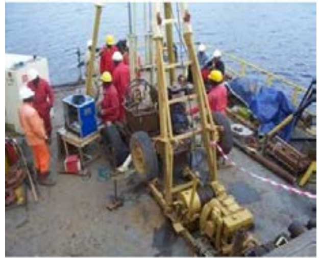
Fig. 4: Geotechnical borehole drilling on water at a near-shore site
