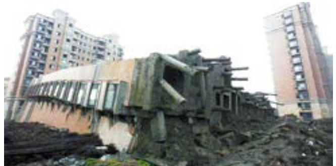
Fig. 1: An example of high-rise building failure caused by defective foundation design
