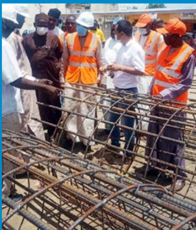
Site inspection after technical meeting
