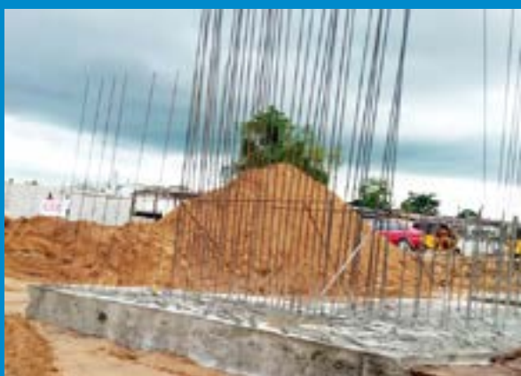
Pile cap and starter bars for pier
