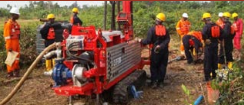
Geotechnical investigation at an SPDC Flow Station
