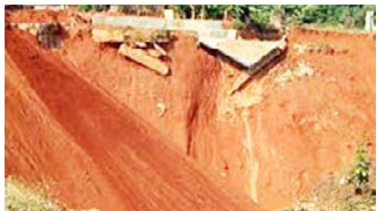
Fig. 3: Landslide destroys 10 houses in Odi, Bayelsa State (Source: Ibid)
