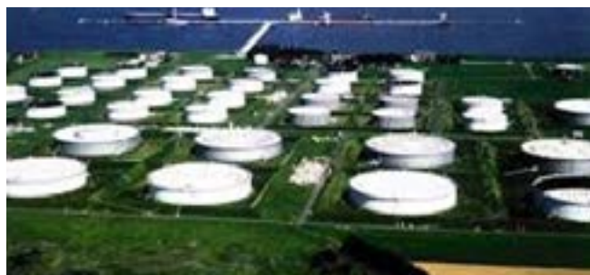
Fig. 5: A petroleum tank farm and terminals on geotechnically modified ground (Source: saratovnetft.com)
