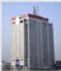
UBA HQ, MARINA, LAGOS 15 Nos. Elevators 25 Stops, 2.5 m/s Completed 2013
