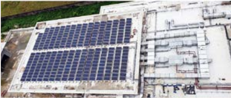
Aerial view of NCDMB 100KW Solar Farm - Electrical / ICT consultancy
