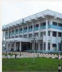
CENTRAL BANK OF NIGERIA ABAKALIKI AND KADUNA 3 Nos. Facade Access Systems Completed 2018
