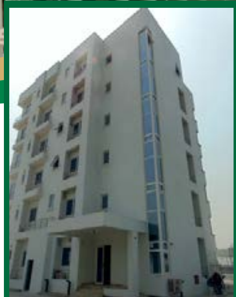
Mechanical Installations for Residential Development at Banana Island
