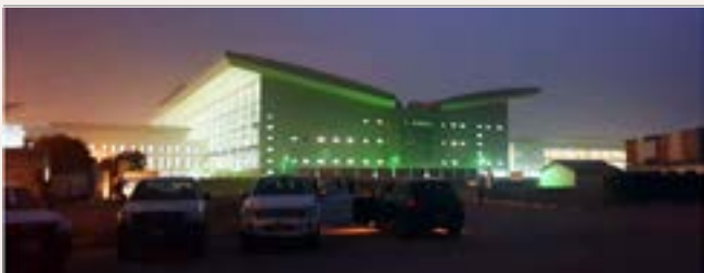
Airport Terminal Building: Abuja and Lagos Airports (similar design for the two) – Electrical/Mechanical consultancy
