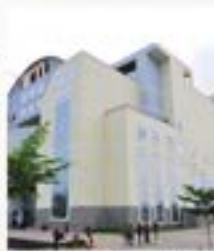
SILVERBIRD GALLERIA, ABUJA 10 Nos. Escalators (with glass side claddings) Completed 2009
