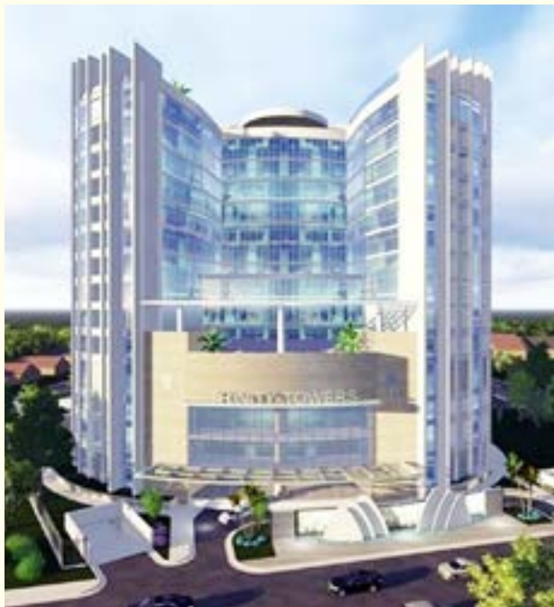
Trinity Towers (Redeemed Christian Church of God) City of David, Oniru, Lagos
