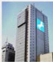
UNION BANK HQ, LAGOS 7 Nos. Elevators 28 Stops, 3.0 m/s with 'DCS' Completed 2015
