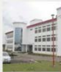
PUNCH NEWSPAPER, MAGBORO 25 Tons DEMAG Crane Completed 2007
