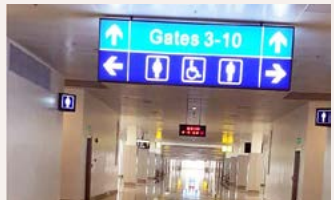
Boarding gate entrance, Abuja Airport - Electrical / Mechanical consultancy
