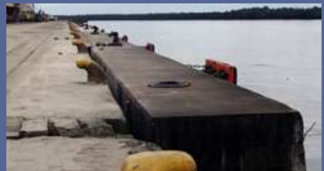
Port Quay Wall Survey: September 2018-January 2018
