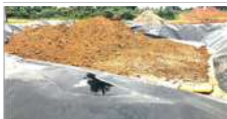
Fig. 15: A mini semi-engineered bio-pile system at Ogoniland, Niger Delta region, Nigeria.
