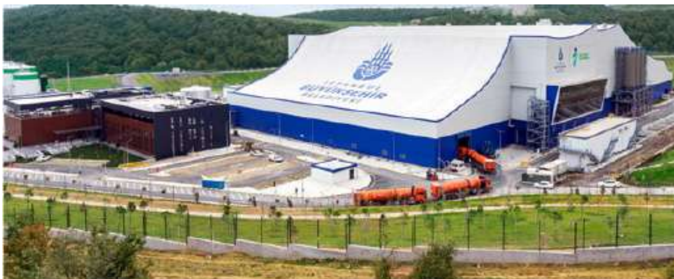
Fig. 1: Istanbul waste power facility. Source: Wikipedia.Org
