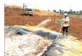
Fig. 17: Irrigating crude oil-contaminated soil after the application of Solpawa® bioremediation products in a mini semi-engineered biocell at Ogoniland, Niger Delta, Nigeria.
