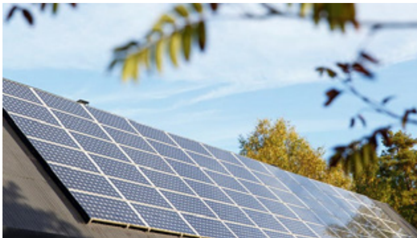
Fig. 3: Bungalow with roof fully covered with solar panels
