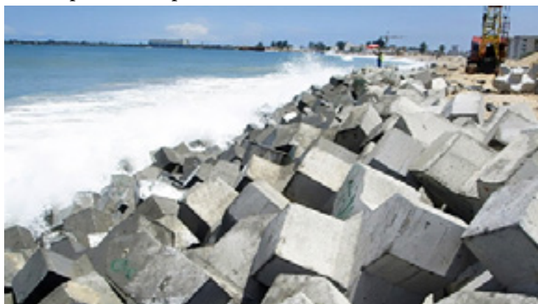
Fig. 7: Nearshore breakwater shore protection
