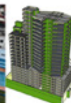
Ocean Heights (Twin tower) in Lagos.
