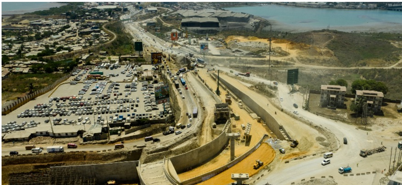
Construction progress at 1 st March 2021
