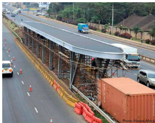
BRT Station under construction opposite Safari Park
