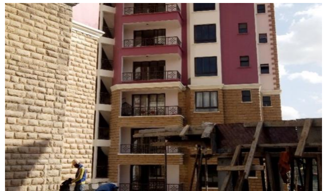
Construction of Serengeti Homes Apartments, Ngong Road
