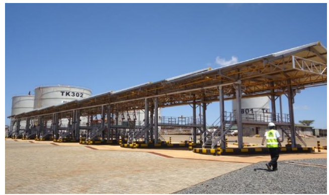
Petroleum Terminal and a Loading gantry at Konza
